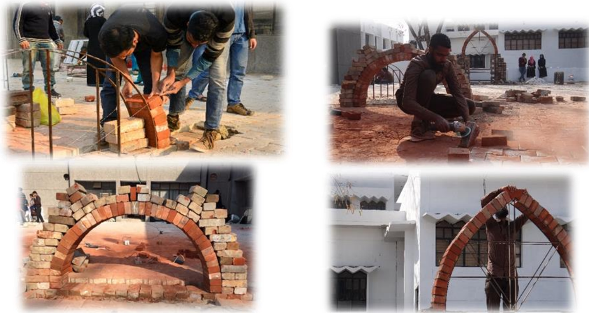
Picture 11-Arch Construction
